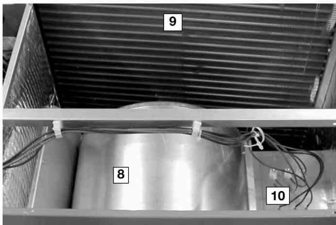
The indoor-section top cover also easily opens to access the removable blower housing and motor (**8**). This also gains total access to the indoor coil for cleaning and service (**9**).
